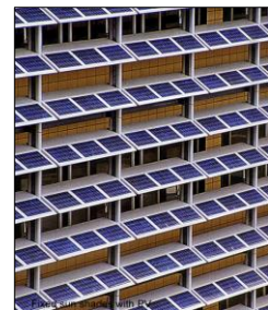
Fig.9: (left, middle) Integration of PV on the sliding sun shading, dwelling houses in Spinnereistraße, Austria, (right) PV used as shading in the Energy Research Centre, Netherlands. (Source: Basnet, 2012)
