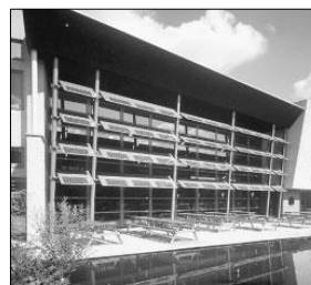
Fig.12: (left) PV shadings as sun protection in the façade, these vertical blinds makes it visually attractive. Design: ABZ Architects, Netherlands. (Kaan, & Reijenga, 2004). (Right) 'Plus-Energie' house, Weiz, Austria. PV used in curved façade adds to the image of the building. Architect: Erwin Kaltenecker, Austria. (Source: Gaiddon et al, 2009)
