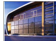
Fig.8: (left) frameless, translucent PV installed in residence home in Calgary, Canada (right) PV integrated into its south glazed façade in Tobias Grau production building in Germany. (Source: https://www.skyfireenergy.com )
