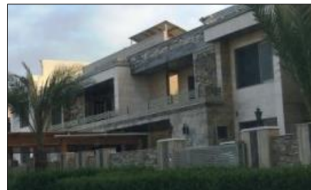
Fig.33: (Example 8-a) (right) Ishtar sweets building, Erbil. Undesirable, added on PV visible on the roof of the building. (Example 8-b- alternative) (left) house with undesirable PV structure in dream city-Erbil. (Source: Researcher)
