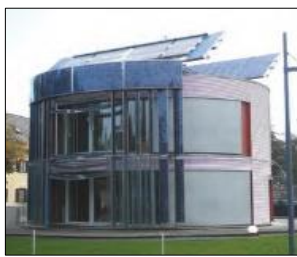
Fig.12: (left) PV shadings as sun protection in the façade, these vertical blinds makes it visually attractive. Design: ABZ Architects, Netherlands. (Kaan, & Reijenga, 2004). (Right) 'Plus-Energie' house, Weiz, Austria. PV used in curved façade adds to the image of the building. Architect: Erwin Kaltenecker, Austria. (Source: Gaiddon et al, 2009)
