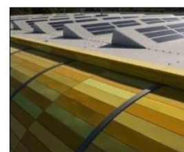
Fig.3: (left) Developed by Lumeta PowerPly, it can be integrated on flat roof, is a part of a fully integrated roofing system (right), Sawtooth roof with PV integration, DIY, Hamburg, Germany. (Source: Basnet 2012)
