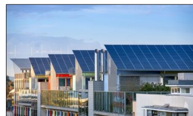
Fig.4: (Left) Integrated PV on the pitched roof of vacation house Bartholomä-Park in Germany (middle & Right) Integrated PV roofs in Schlierberg Solar Settlement housing estate in Freiburg, Germany. (Source: Basnet 2012)
