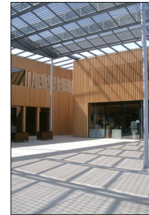
Fig.6: (Left) PV samples for skylight in different colors & textures, (middle & right) Atrium with PV modules, Ludesch/Vibg., Austria. (Source: tps://solarintegrationsolutions.org )
