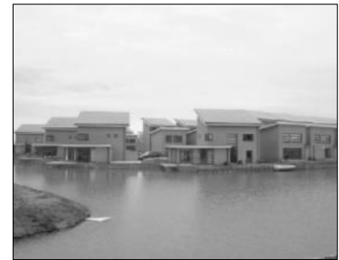
Fig.11: (left) J-House, Tokyo, Japan. Natural integration of the PV system in the building. Architect: Jiro Ohno, (right) The dwellings at the 5 MW project in the HAL district, Langedijk, Netherlands. It has a large PV roof without any perforations. This strengthens the architectural expression of the roof design. Source: (Gaiddon et al, 2009)
