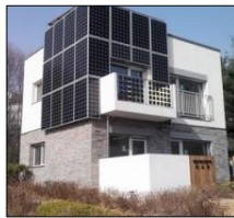
Fig.7: (left) bronze and gold colored PV cells used in the "home+" building project, tuttgart, Germany, (right) PV integrated into the opaque parts of house in Seoul, South Korea. (Source: Basnet, 2012)
