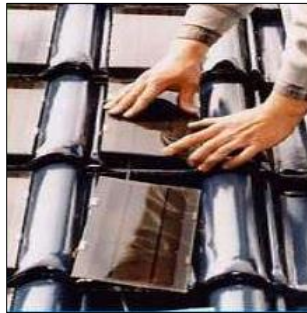
Fig.5: (left) Roof with integrated PV tiles, (right) PV shingles. (Source: Basnet 2012)
