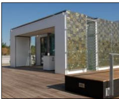
Fig.7: (left) bronze and gold colored PV cells used in the "home+" building project, tuttgart, Germany, (right) PV integrated into the opaque parts of house in Seoul, South Korea. (Source: Basnet, 2012)
