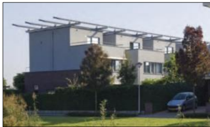
Fig.17: Single-family houses 'De Keen', Etten-Leur, The Netherlands. The application of PV has led to a new architectural concept. Architect T. H. Reijenga, BEAR Architekten. (Source: Gaiddon et al, 2009)
