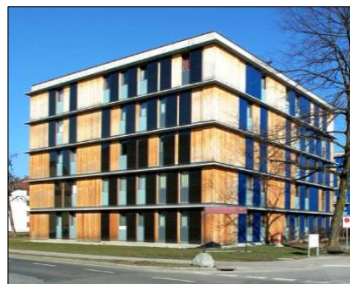
Fig.9: (left, middle) Integration of PV on the sliding sun shading, dwelling houses in Spinnereistraße, Austria, (right) PV used as shading in the Energy Research Centre, Netherlands. (Source: Basnet, 2012)
