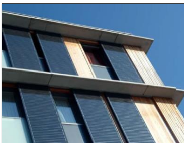
Fig.9: (left, middle) Integration of PV on the sliding sun shading, dwelling houses in Spinnereistraße, Austria, (right) PV used as shading in the Energy Research Centre, Netherlands. (Source: Basnet, 2012)
